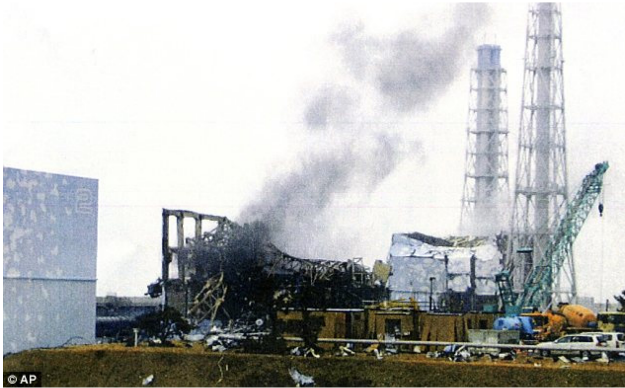
Smoke: Fresh safety concerns arose today as black smoke was spotted emerging from Unit 3 of the plant, prompting a temporary evacuation of all workers from the complex
