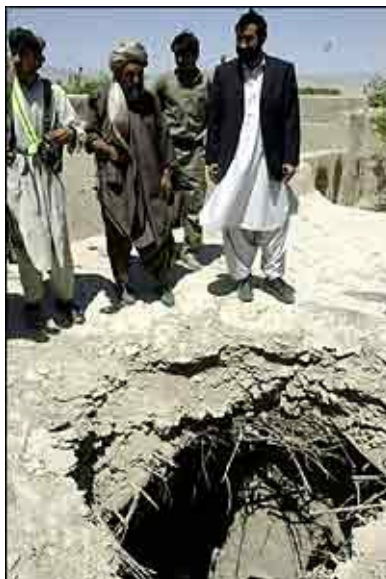
Bomb damage was widespread
