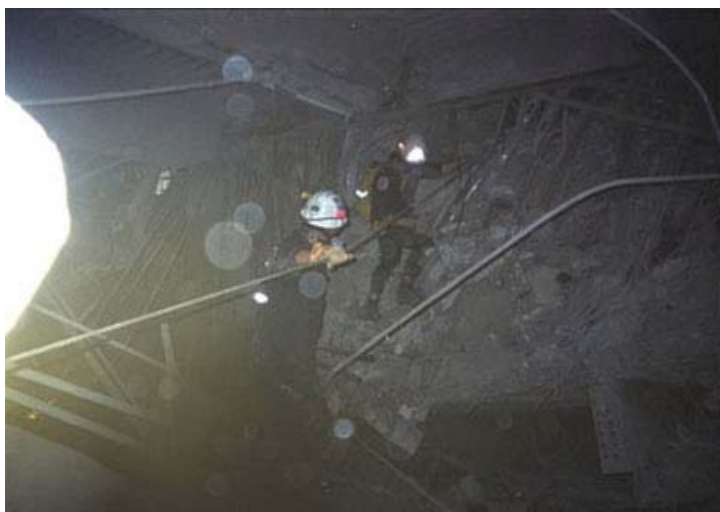
Approaching the entrance to the sub-level areas of Building 6
