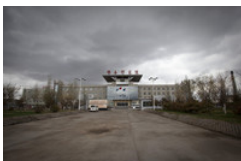
The research facility at Inner Mongolia Baotou Steel Rare-Earth Hi-Tech Co. Photographer: Nelson Ching/Bloomberg
