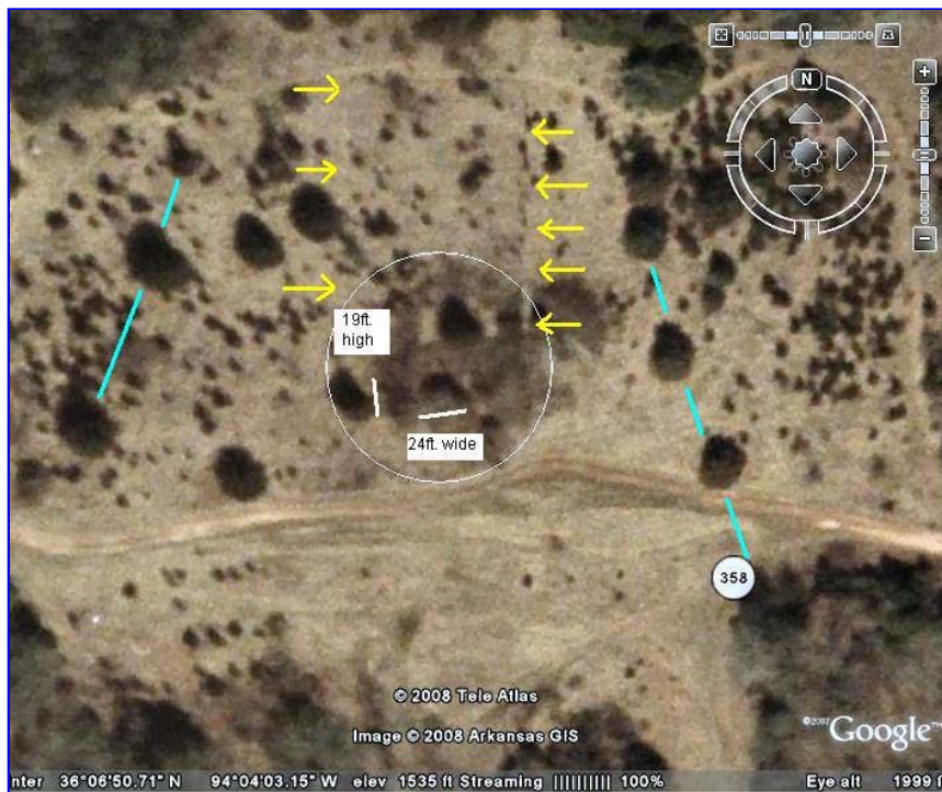
Fig 5 – White circle shows a close-up of a tunnel entrance (Fig. 4.) With an opening 19ft. high and 24ft. wide a tractor trailer could easily drive inside. This image is from an elevation of 1,999ft. From this elevation we see that this tunnel is much larger than it appears here.
