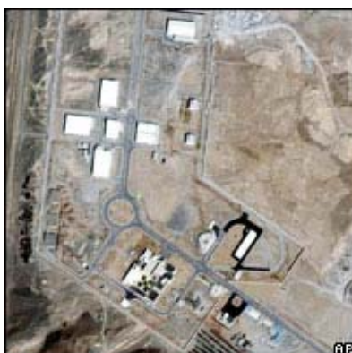
The Natanz plant is buried under concrete, metal and earth
