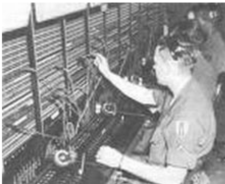
Military Switchboard, 1966, in Saigon
