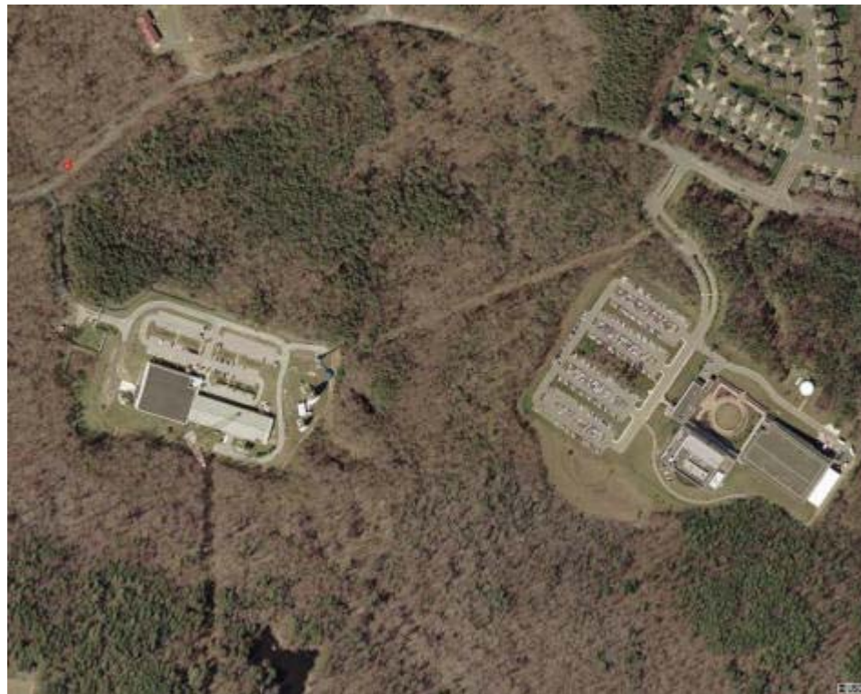
Covert eavesdropping of European cell phone calls involve these two facilities located on Federal property between Laurel and Beltsville, Maryland: the State Department's Diplomatic Telecommunications Service (l.) and the NSA-CIA Special Collection Service (r.).
