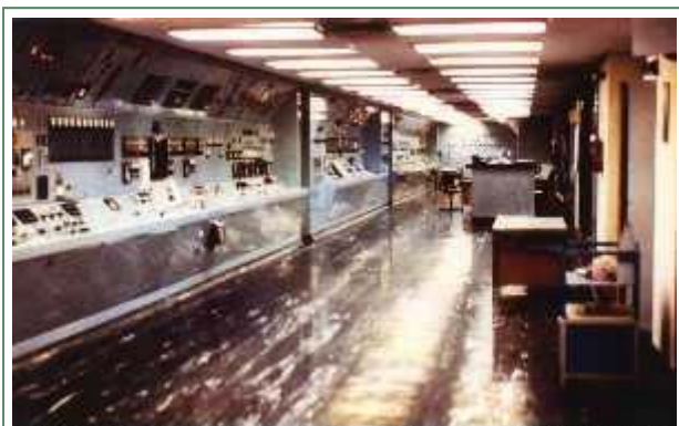
Control room of Israel's plutonium separation plant at Dimona. Photo by Mordechai Vanunu.
